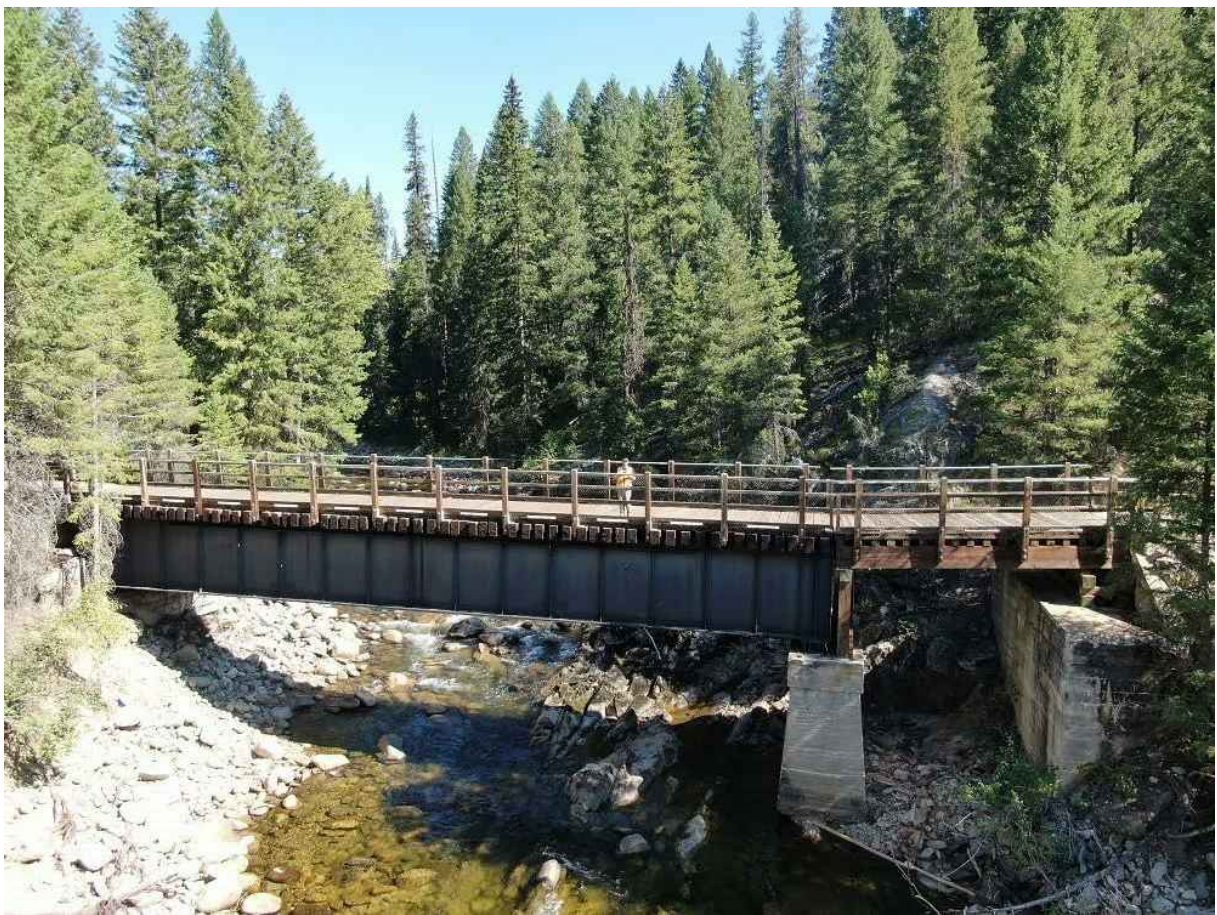
PHOTO 2: OVERVIEW OF BRIDGE LOOKING UPSTREAM
